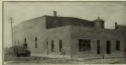
FIG. 1. STATION OF LEBANON HEATING COMPANY
